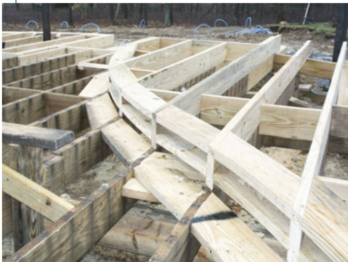
Figure 8. The upper deck meets the lower deck in a sinusoidal compound curve, which is supported by a complex blocking system (below).
