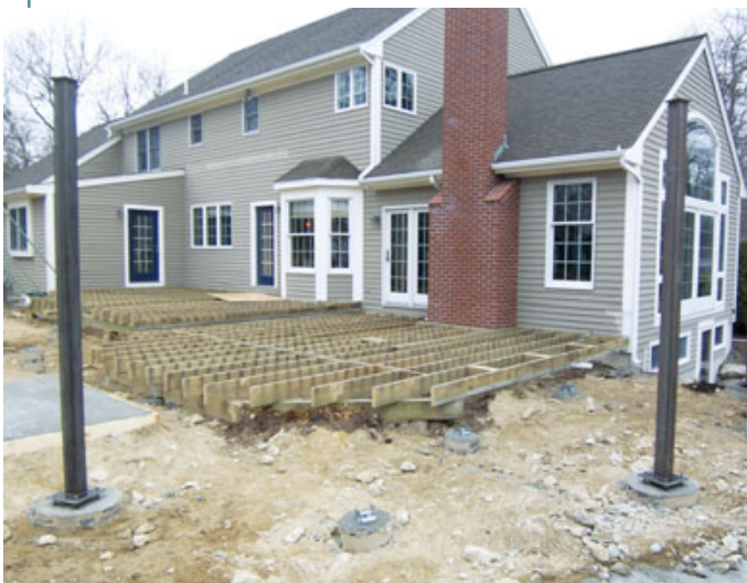
Figure 6. The fruit of the computer-drawn plans was correctly located footings for both the deck and the curved pergola.
