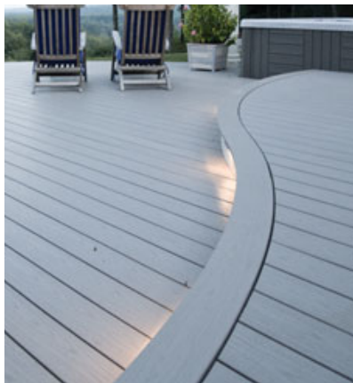
Figure 8. The upper deck meets the lower deck in a sinusoidal compound curve, which is supported by a complex blocking system (below).
